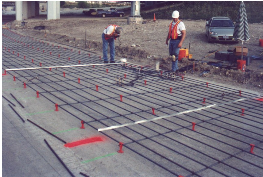
Figure 87. Instrumented section delineated by crack inducers.
