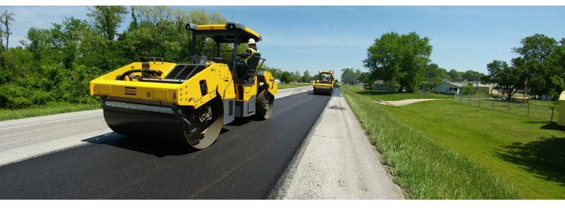
The Missouri Department of Transportation (MoDOT) executed a year-long project throughout 2017 to demonstrate the use of intelligent compaction (IC), infrared scanning (IR), and Veta software to improve pavement construction operations.
