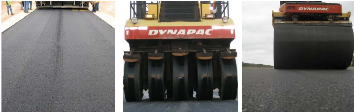
Figure 6 – Streaking from poor paving practice (a) and pneumatic (b) and steel drum (c) compaction
