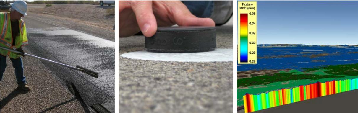
Figure 3 – Constructing undesired texture (a), measuring with sand patch (b), managing pavement texture (c)
